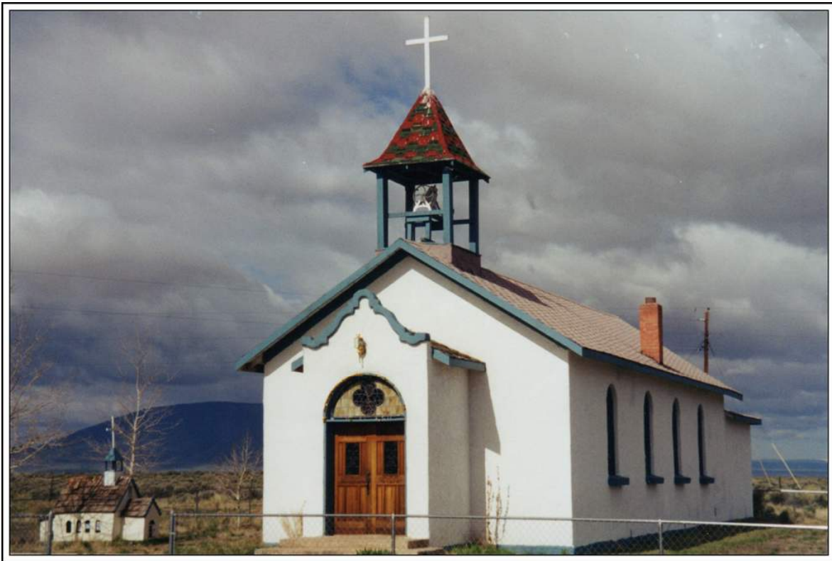
An active church building at the site of Manzanares, Colorado Note the small model of the building at the lower left of the photograph. Photograph by William H. Bauer May 11, 1999
