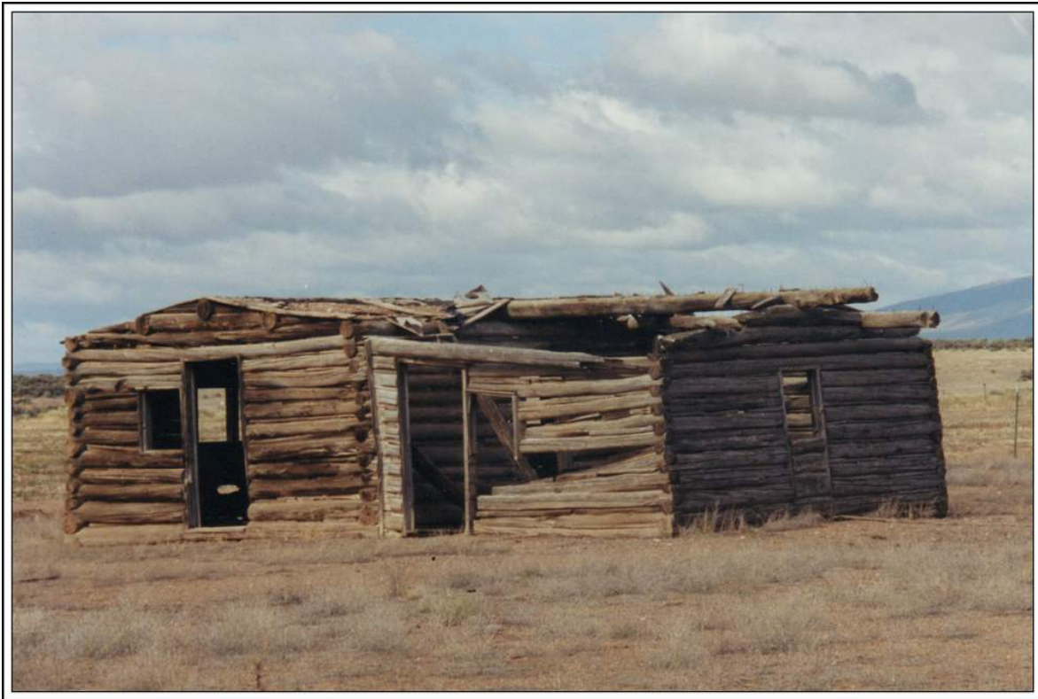
Abandoned log building at the site of Eastdale, Colorado Photograph by William H. Bauer May 11, 1999
