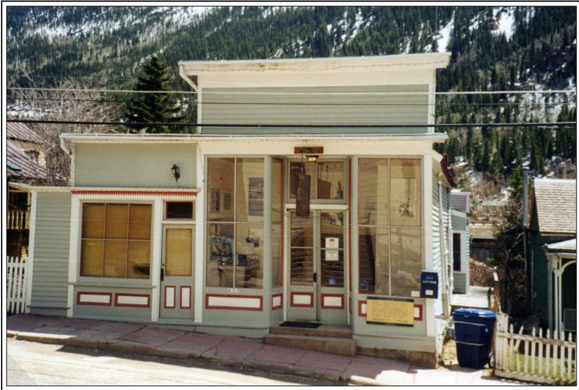
Post Office – Silver Plume, Colorado Photograph by William H. Bauer May 10, 1998
