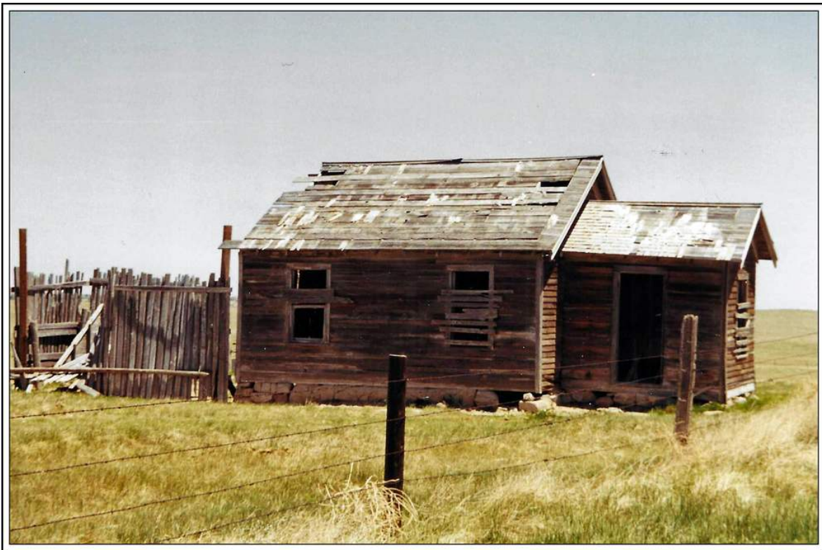
Abandoned building at the 1898 site of Avalo, Colorado
