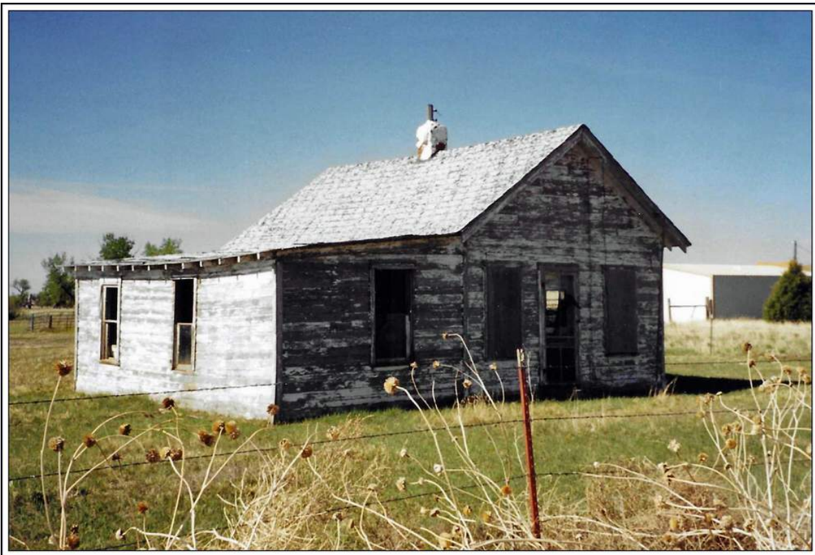
Abandoned building at site of Cornish, Colorado Photograph by William H. Bauer May 18, 1998
