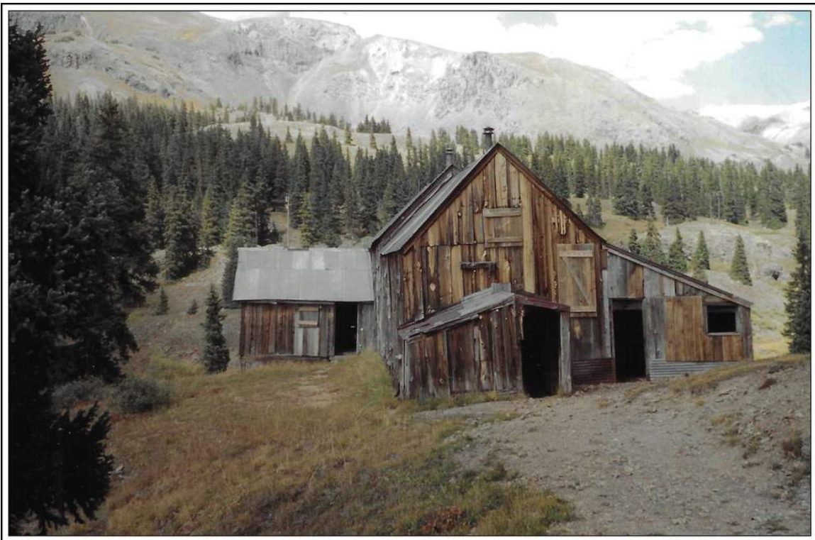
Congress, Colorado – Abandoned buildings along south side of US Highway 550, near the summit of Red Mountain Pass
