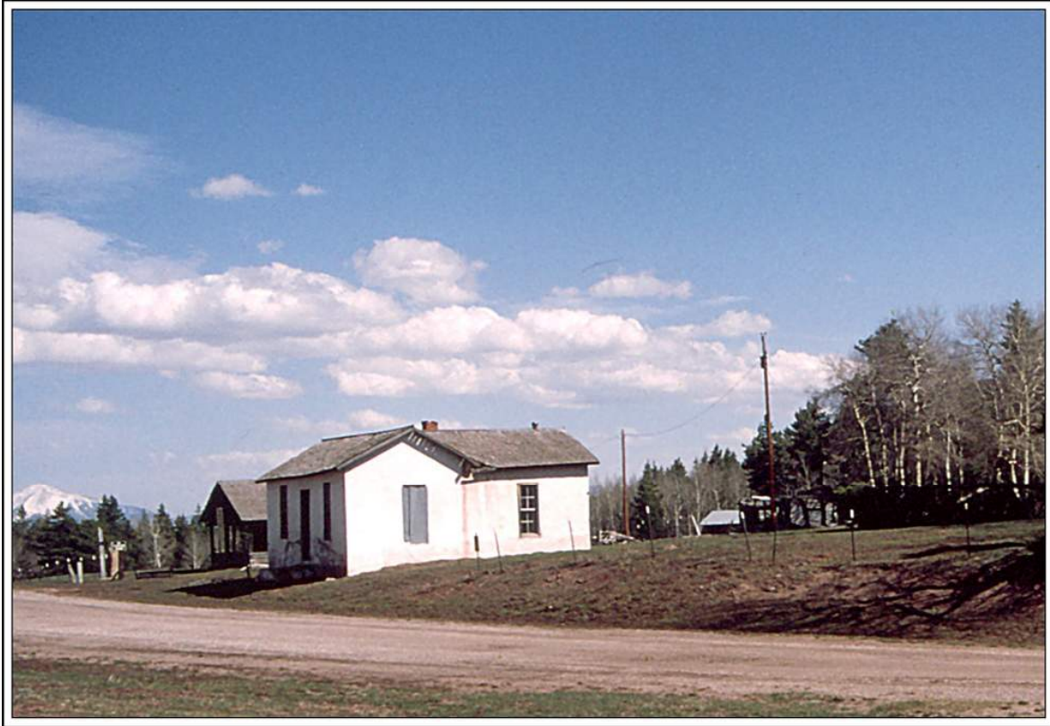
One of the remaining buildings at Veta Pass, Colorado. This building may have been the railroad station at the pass. Photograph by James L. Ozment May 18, 1999
