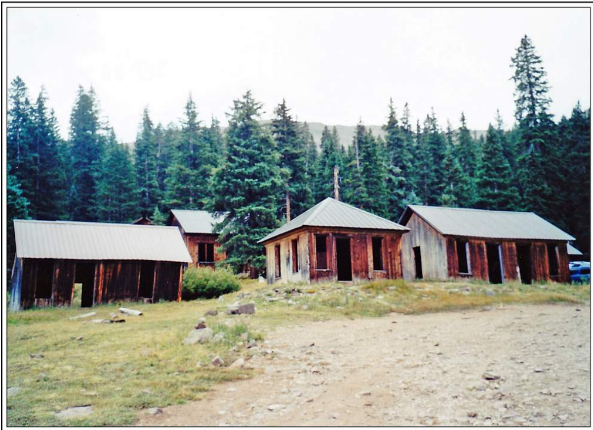
Stabilized buildings at the second site of Carson Photograph by William H. Bauer September 5, 2001
