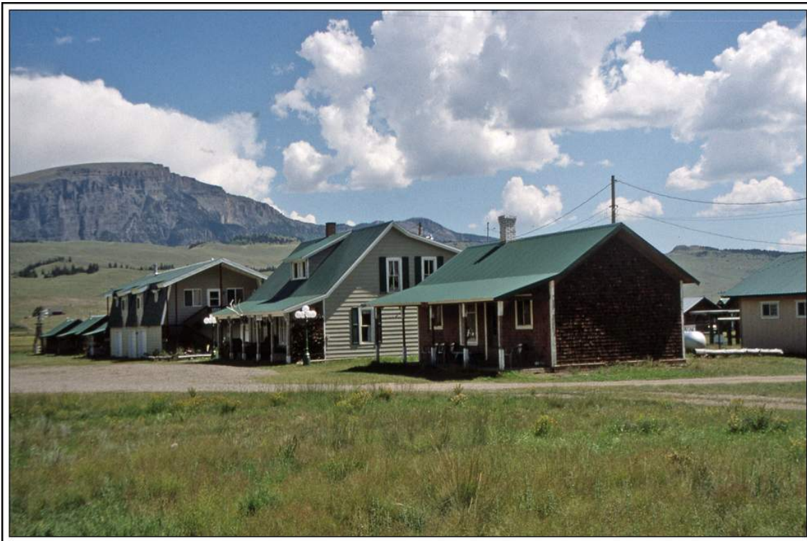
The San Juan Guest Ranch, final location of the San Juan Post Office. The building on the right was the stage station.
