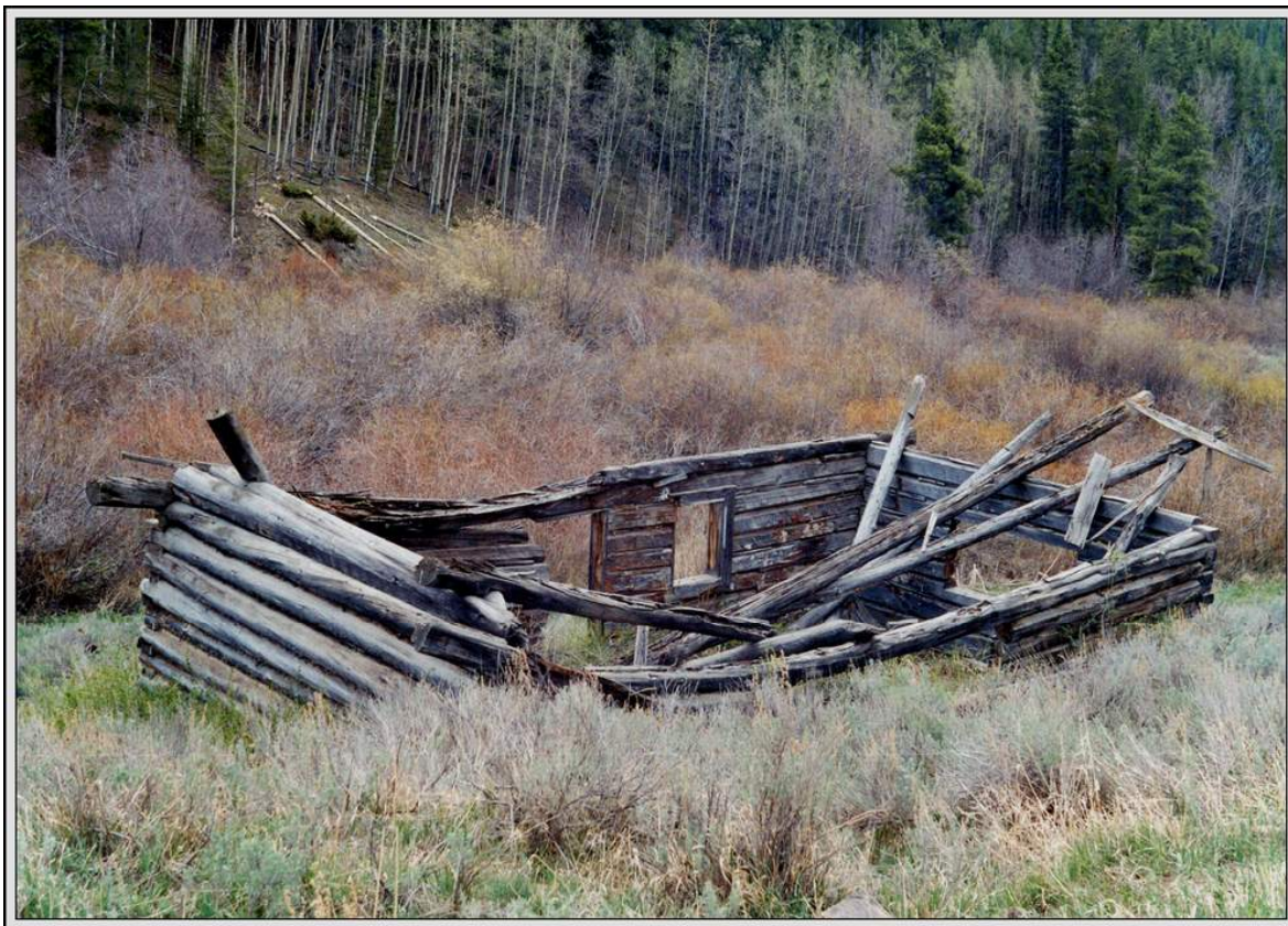
Remnants of one of the cabins at Bowerman, Colorado Photograph by James L. Ozment May 2002
