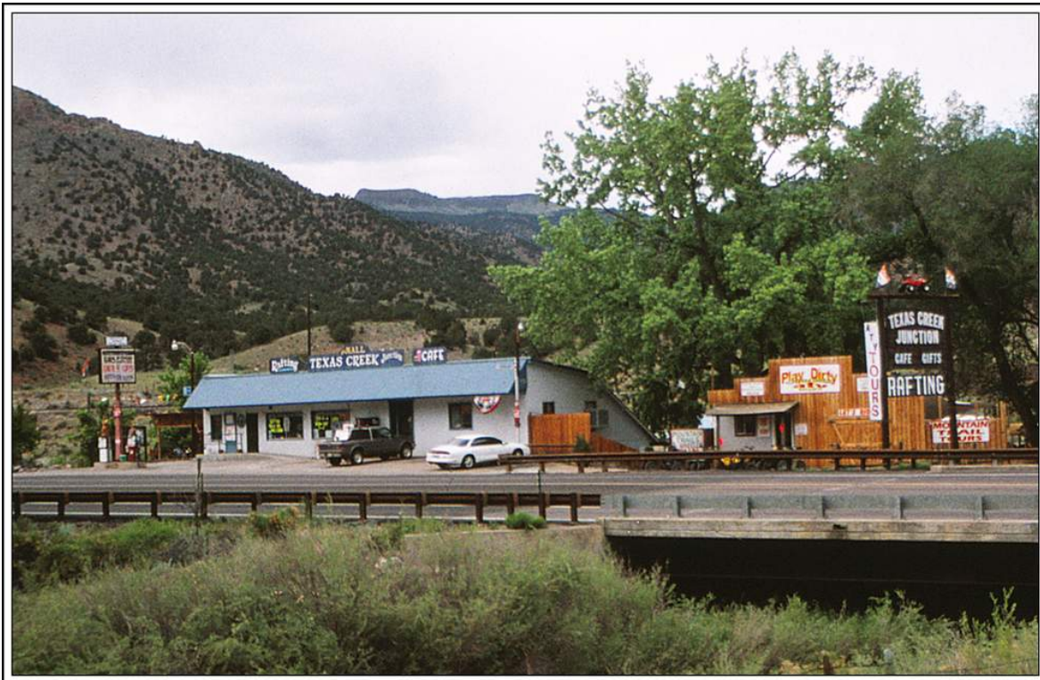
Texas Creek, Colorado – Overview looking north across US Highway 50 Photograph by James L. Ozment May 23, 2001
