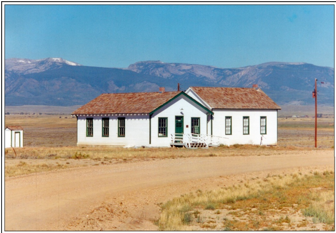
The Community Building, Coalmont, Colorado Photograph by William H. Bauer September 15, 1998
