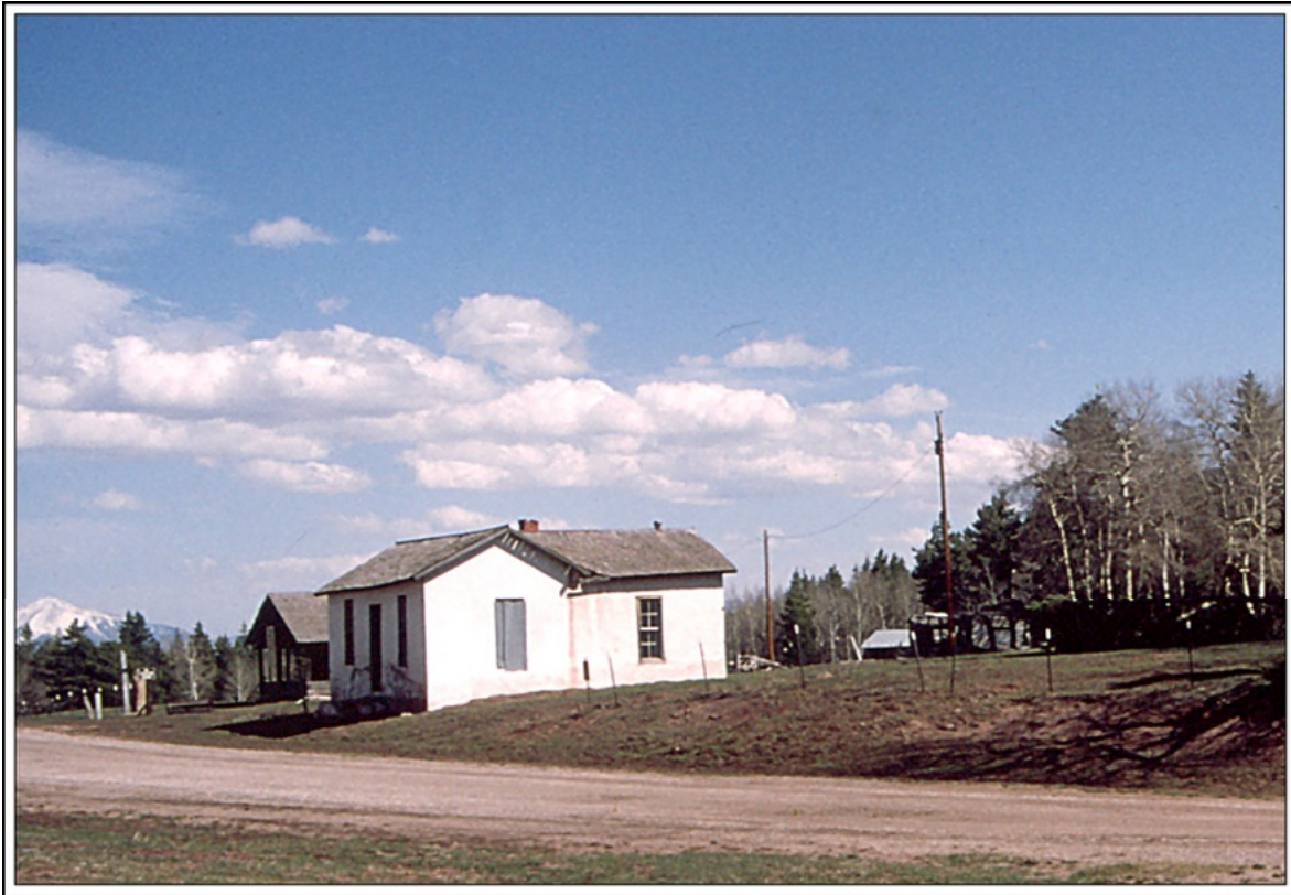
One of the remaining buildings at Veta Pass, Colorado. This building may have been the railroad station at the pass. Photograph by James L. Ozment
