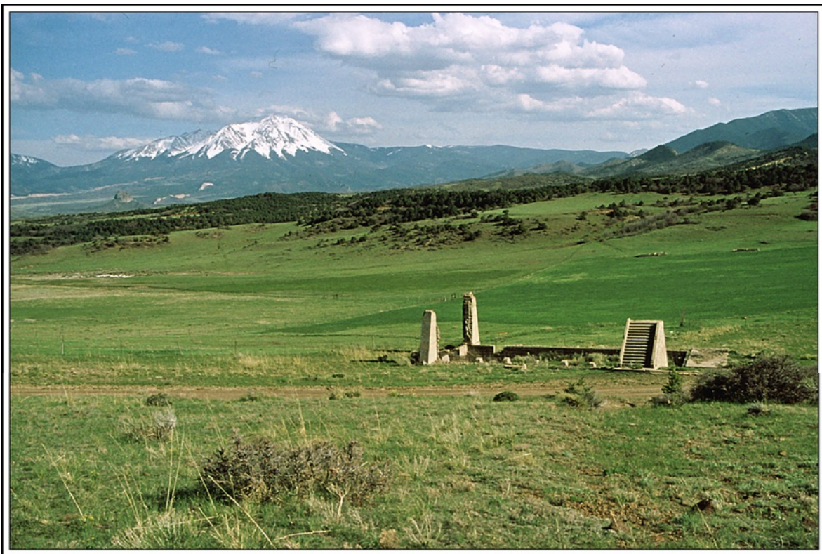
Site overview and building remnants at Oakview, Colorado Photograph by William H. Bauer May 18, 1999
