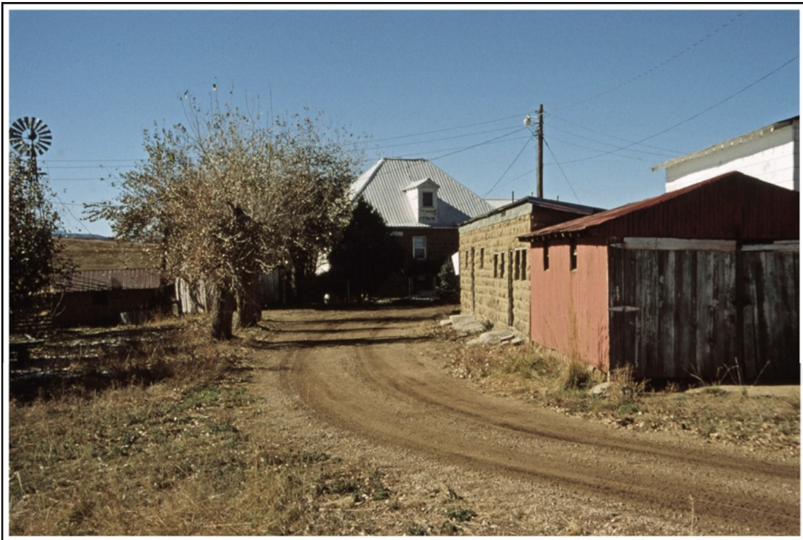
Ranch buildings at the site of Scissors and Capps Photograph by William H. Bauer October 30, 1999
