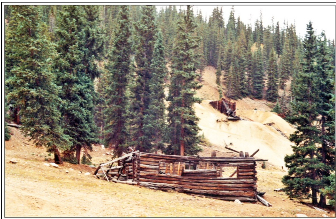
Building ruins and mine dump at site of Drew, Colorado
