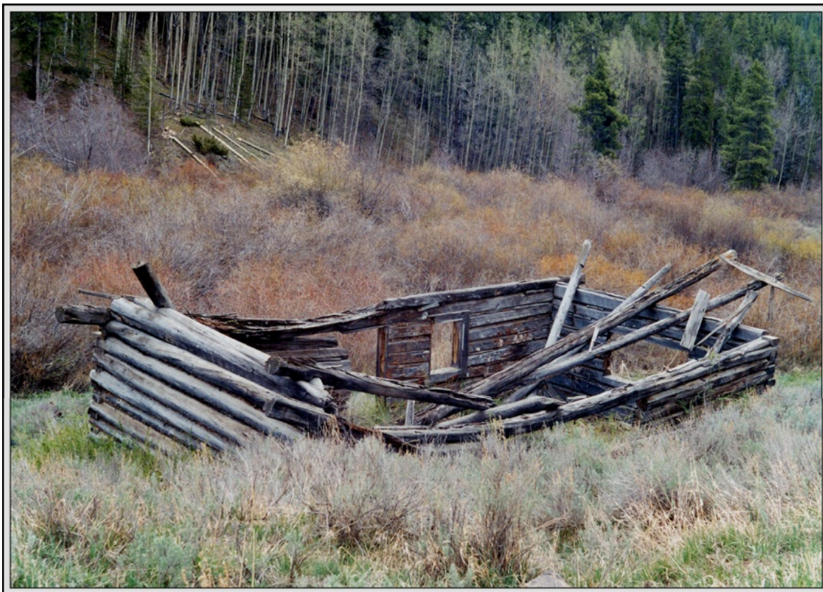
Remnants of one of the cabins at Bowerman, Colorado Photograph by James L. Ozment May 2002
