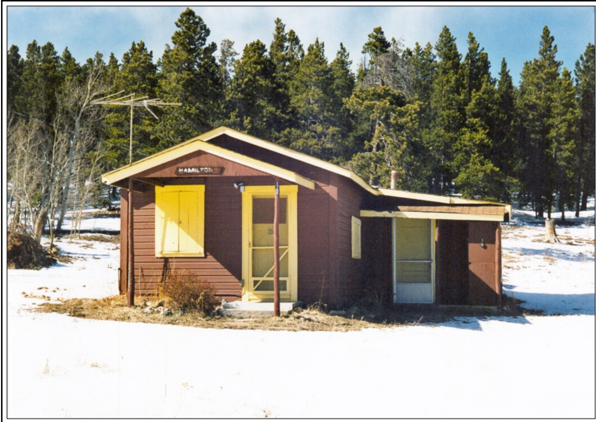
Gilpin, Colorado: Log cabin restored for use as a summer residence Photo by James L. Ozment April 5, 1998
