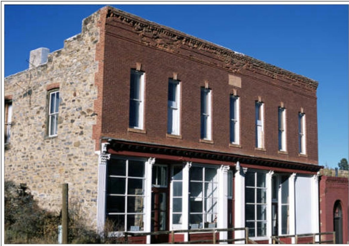
The Masonic Hall in Nevadaville, Colorado – A meeting is held in this building once each year
