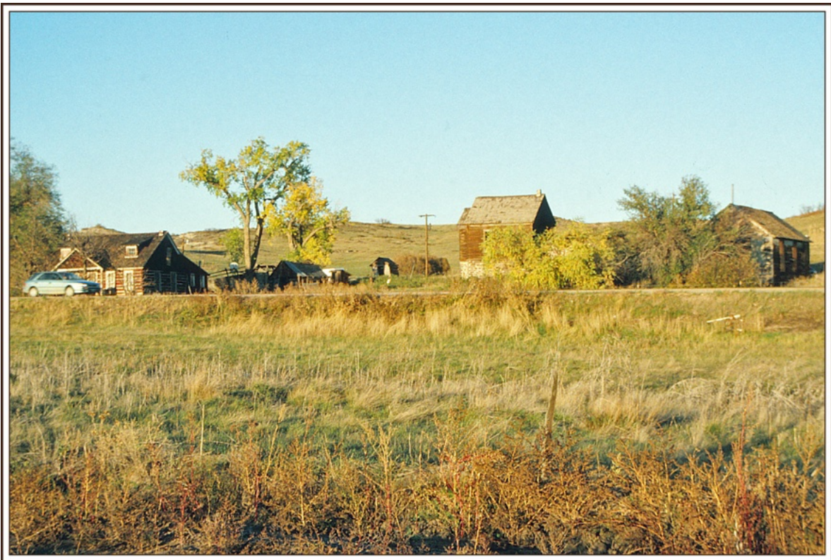
Keystone – Ranch/Buildings Overview
