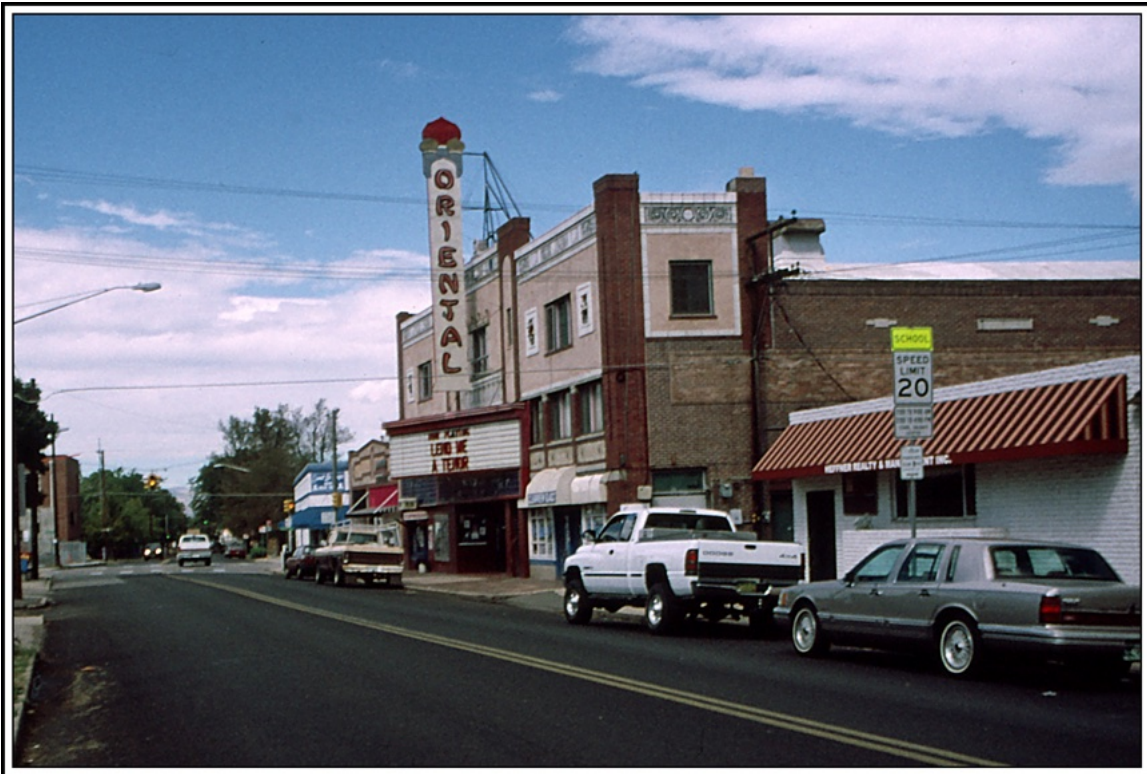
Alcott community – Street scene looking west from the corner of West 44th Avenue and Stuart Street.
