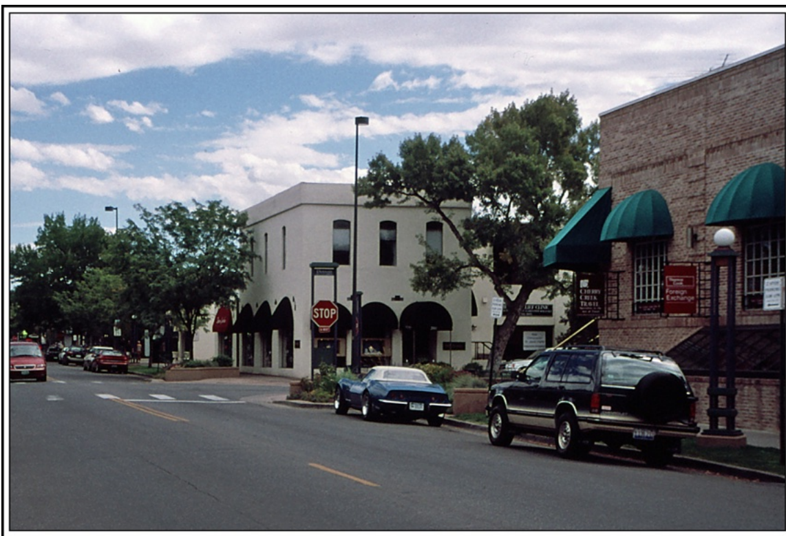
1901 location of the Harman Post Office on the southeast corner of East 3rd Avenue and Detroit
