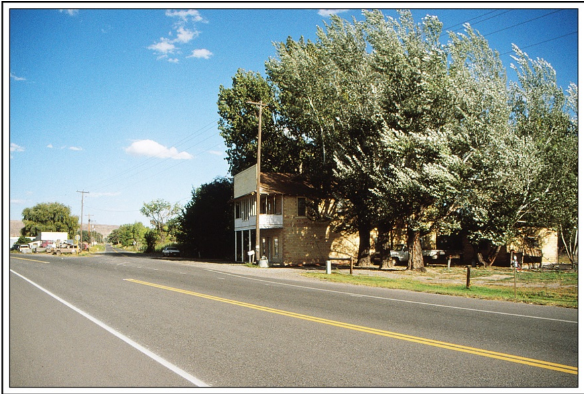
Read, Colorado – Junction of Colorado Highway 92 and County Road H75 Photograph by William H. Bauer September 22, 2000
