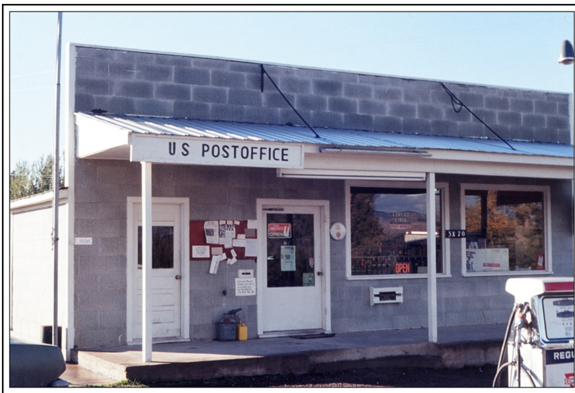
Cory, Colorado — Cory General Store and Post Office Photograph by W. H. Bauer September 22, 2000
