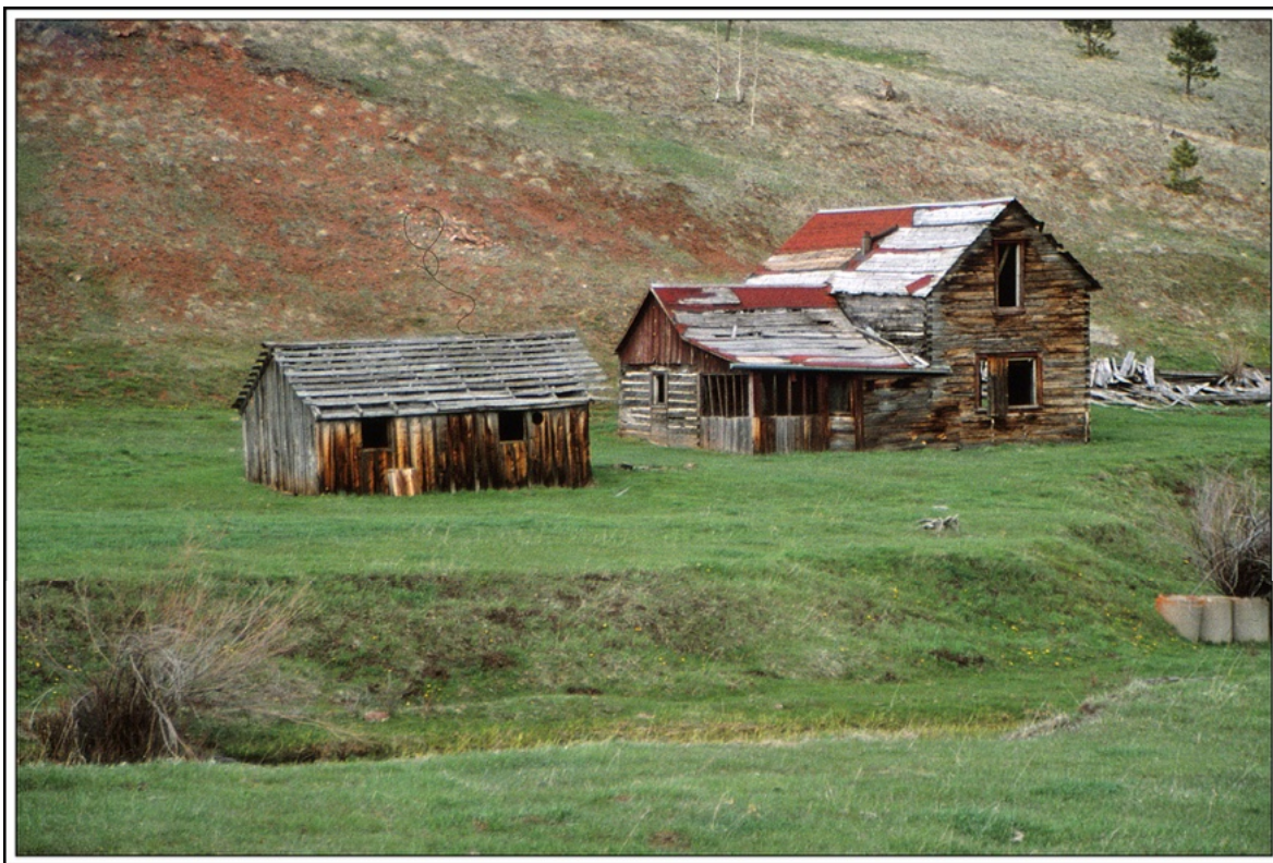
Abandoned ranch buildings at the site of Forestdale, Colorado Photograph by William H. Bauer May 19, 1999
