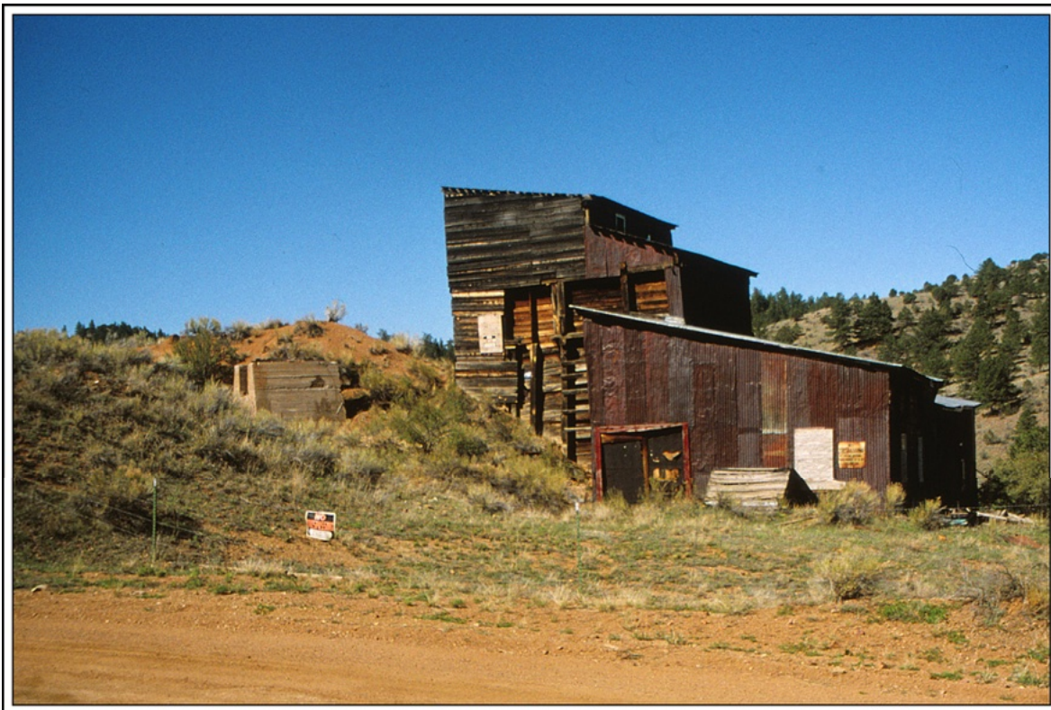
Ilse, Colorado – Remaining mine or mill buildings near the community Photograph by William H. Bauer May 23, 2001
