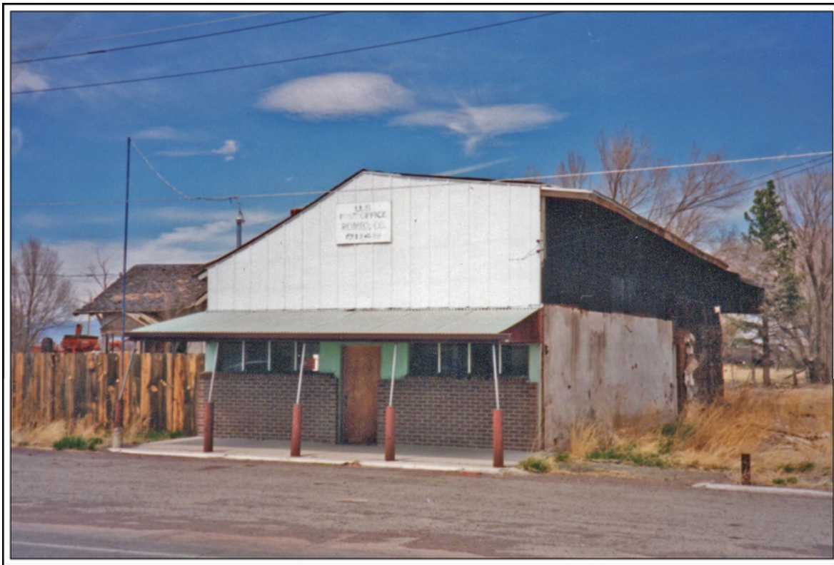
The old post office building at Romeo, Colorado Photograph by James L. Ozment May 4, 1997
