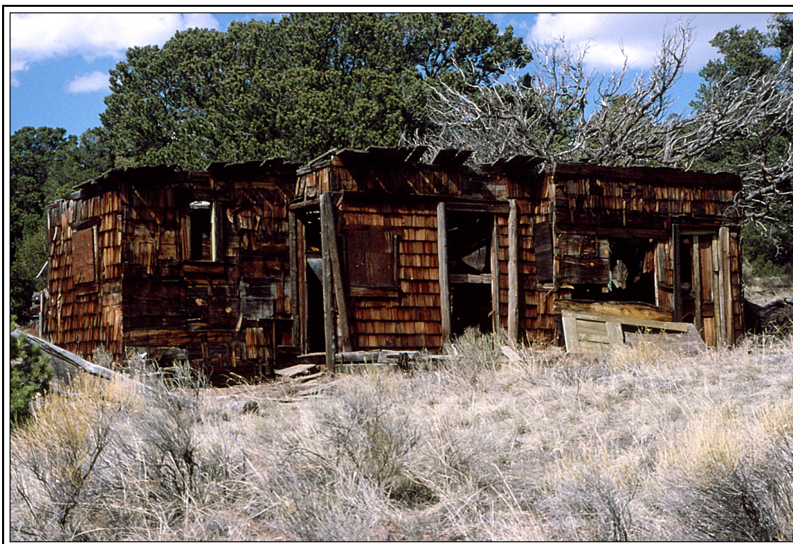
Abandoned building at the site of Montville, Colorado, within the boundaries of the Great Sand Dunes National Park. Photograph by William H. Bauer May 8, 1999
