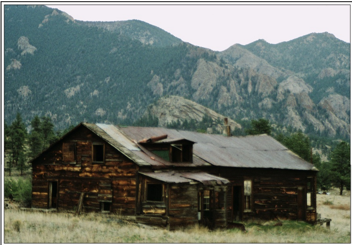
Abandoned building at Tarryall – This building may have been a store and possibly the post office. Photograph by William H. Bauer May 17, 2004
