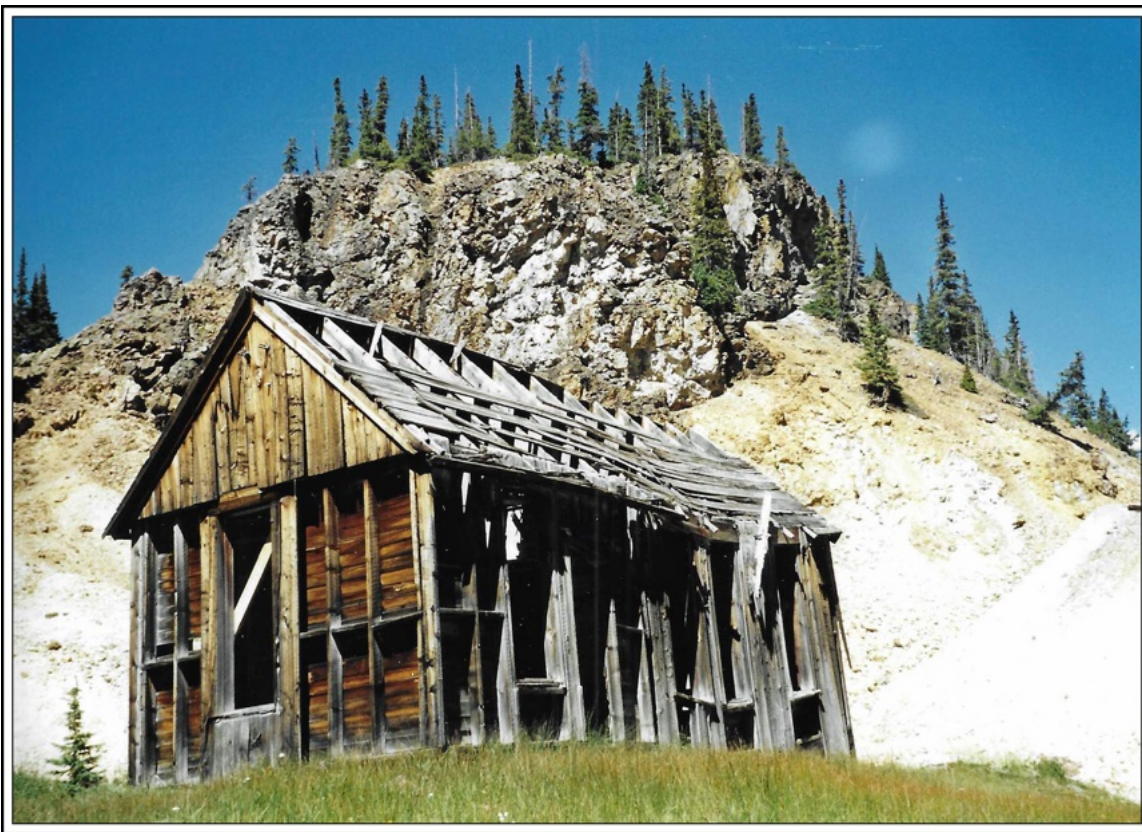
The remaining building of the National Belle Mine at Red Mountain, Colorado Photograph by William H. Bauer August 25, 2004
