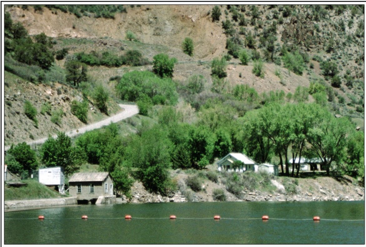
View of River Portal, Colorado and the road that descends to the Gunnison River in the Black Canyon of the Gunnison National Park
