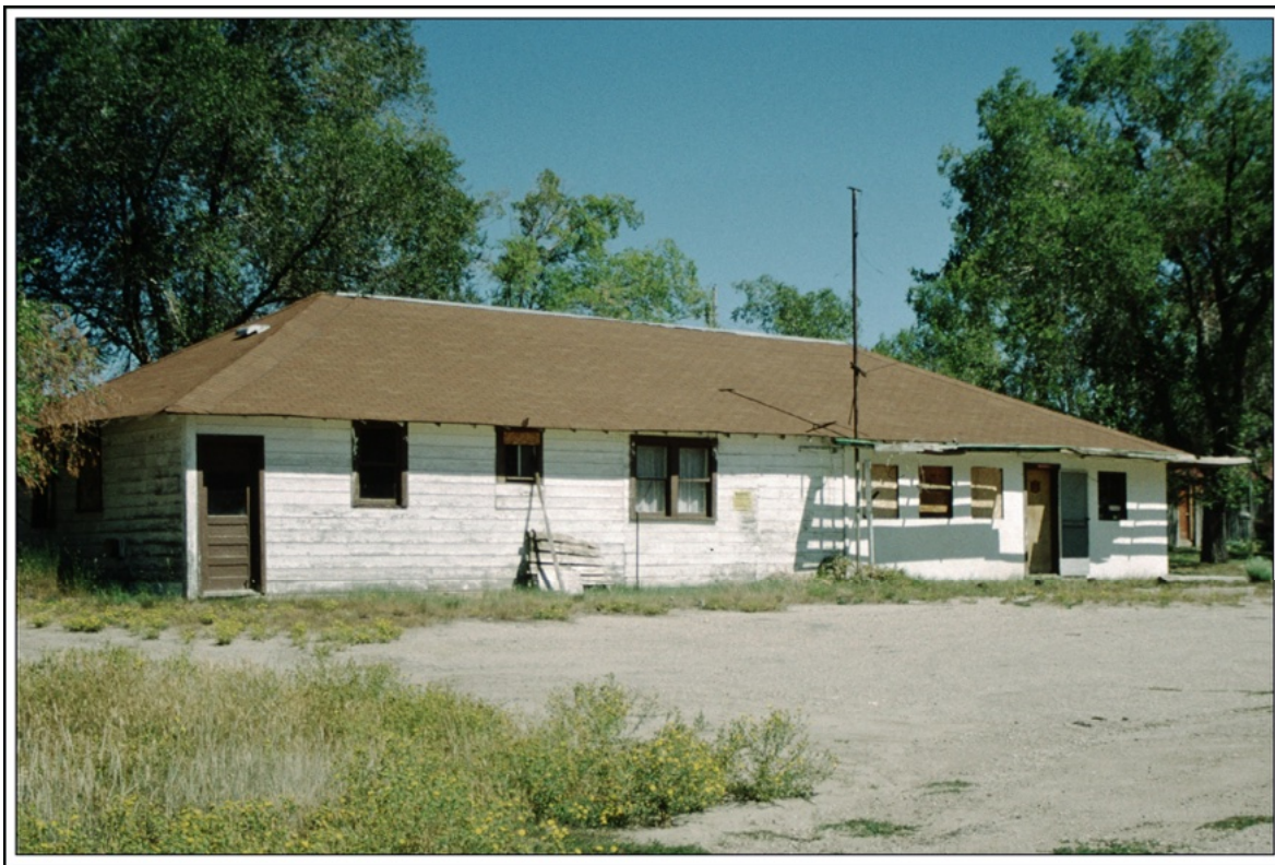
This building once housed the Elk Springs Community Post Office and a café. Photograph by W. H. Bauer September 2, 1998
