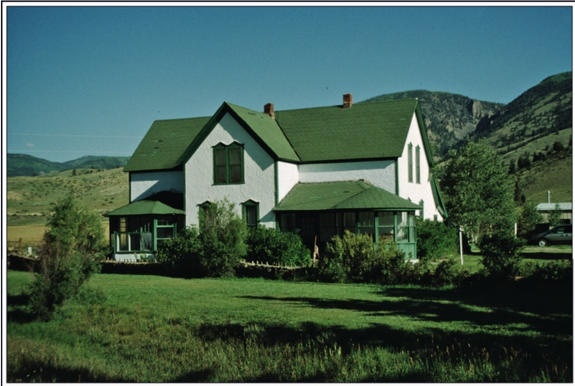
Wason, Colorado – One of the main buildings of the guest ranch at the site of Wason Photograph by William H. Bauer September 4, 2001
