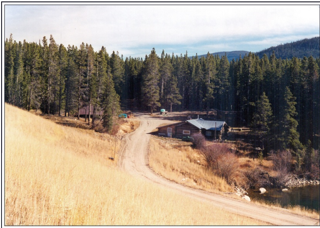
Buildings below the dam at the west end of Chambers Lake Photograph by James L. Ozment October 27, 1999
