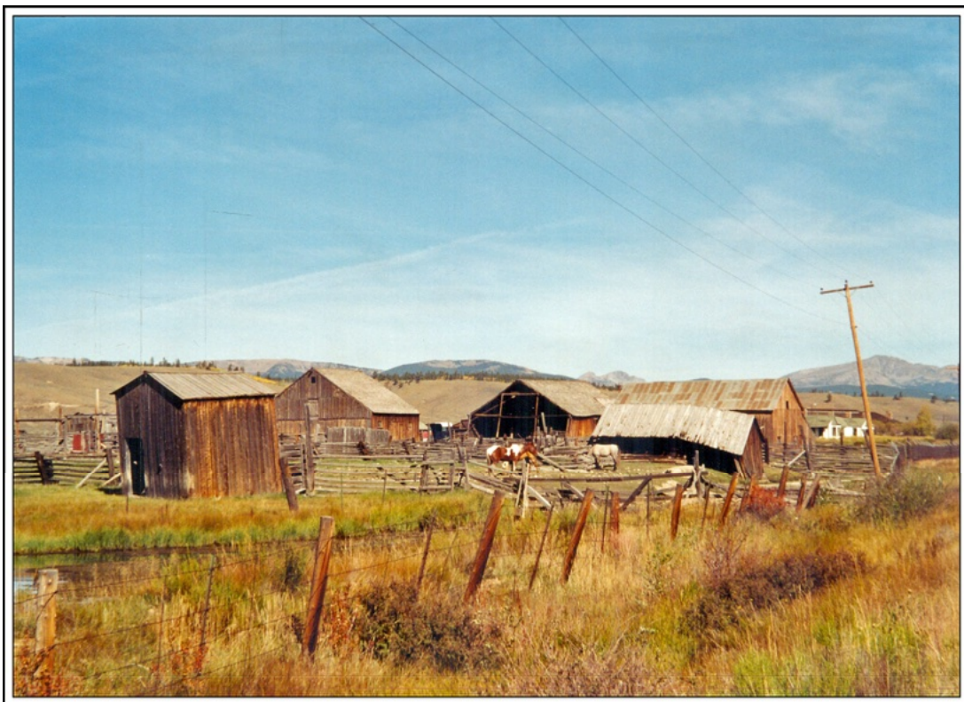
Ranch buildings on the west side of US 24 at site of Hope (Snowden) near Kobe Siding Photograph by William H. Bauer September 13, 2000
