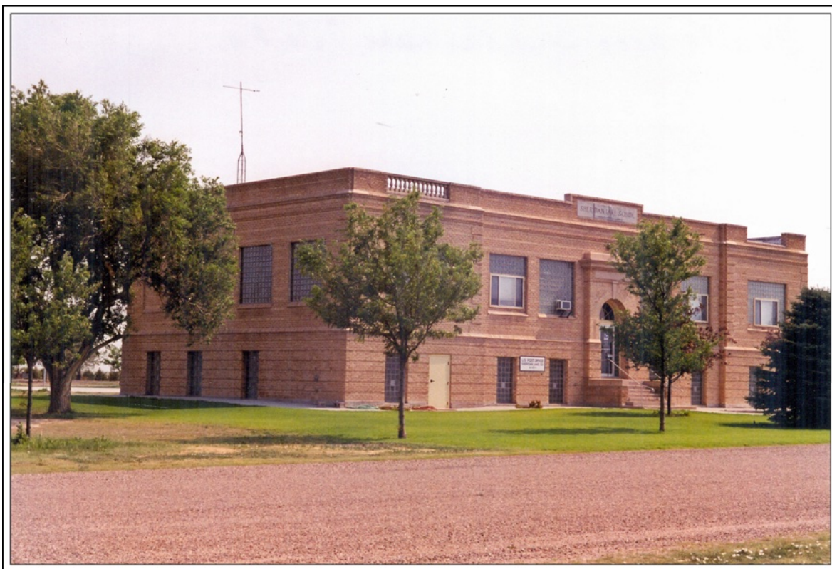
Sheridan Lake, Colorado The post office is located in the former Sheridan Lake School Building. Photograph by James L. Ozment
