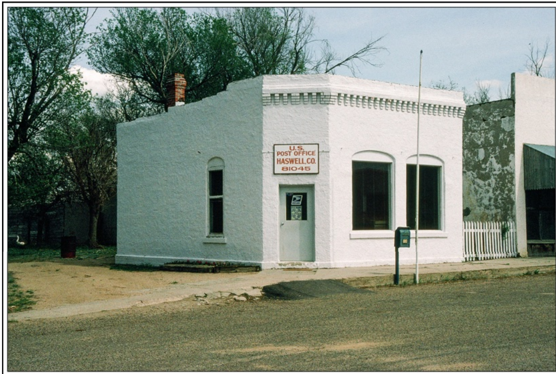
Post Office building, Haswell, Colorado Photograph by W. H. Bauer May 12, 1997
